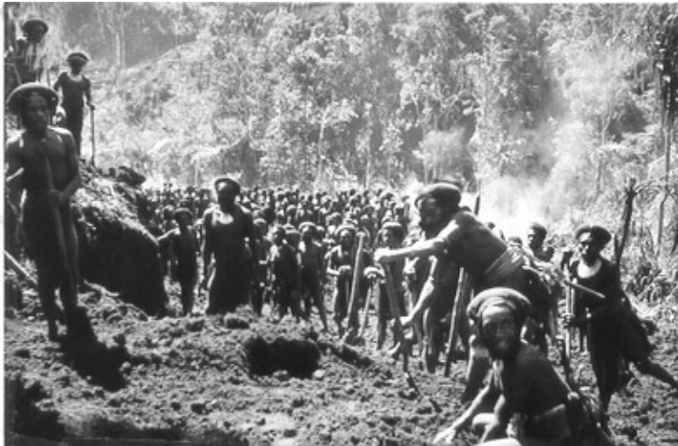
Figure 1. Kewa men working on the Ialibu-Kagua road (July 1960).
